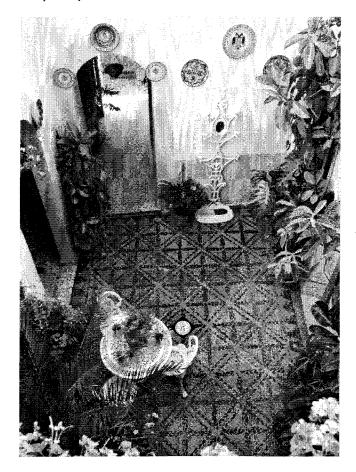
Fig. 3. Black and white pebbles, set in a porous mortar, can be wetted repeatedly during hot weather for nearly continuous evaporative cooling. Cordoba, Spain, Calle Zarco. From John S. Reynolds, Courtyards: Aesthetic, Social, and Thermal Delight (New York: John Wiley and Sons, 2002; page 35.)
